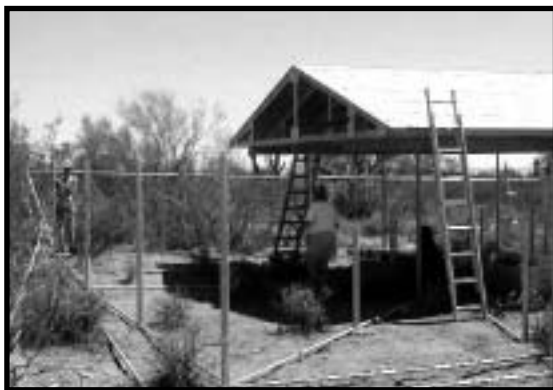
Pen "A" Under Construction
