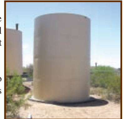
New Water Tank
